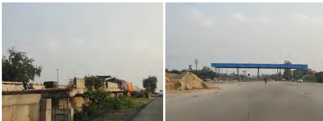
Figure 4-5 ROB & Toll Plaza under construction
