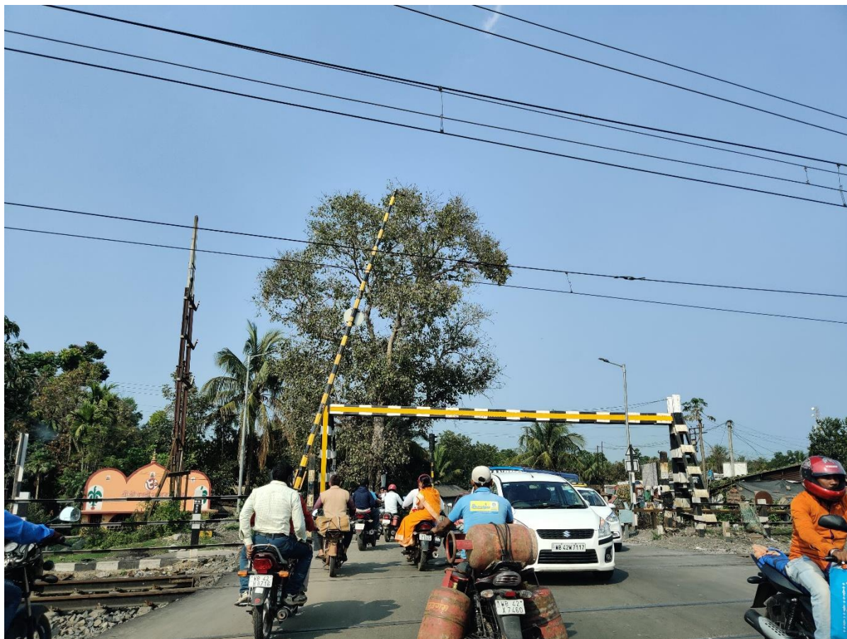
Figure 4-3 Railway level crossing at GT road
