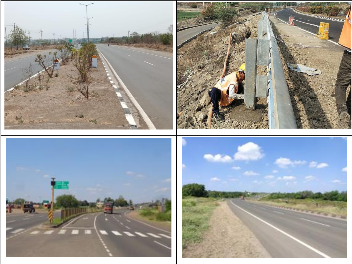
Figure 2-2: Photographs showing Project Corridor
