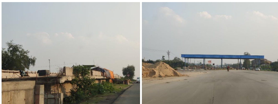
Figure 4-5 ROB & Toll Plaza under construction
