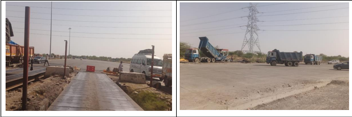
Figure 2-2 : Photographs showing Project Corridor
