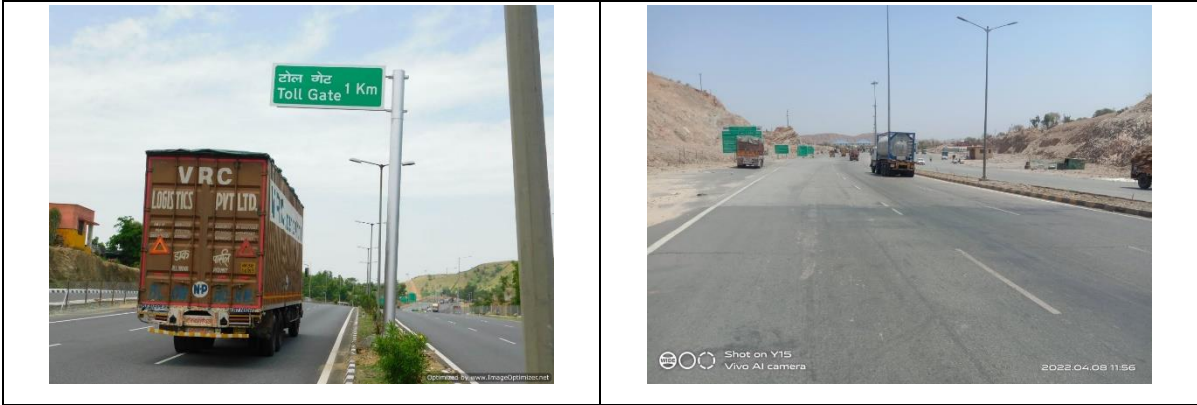
Figure 2-2 : Photographs showing Project Corridor
