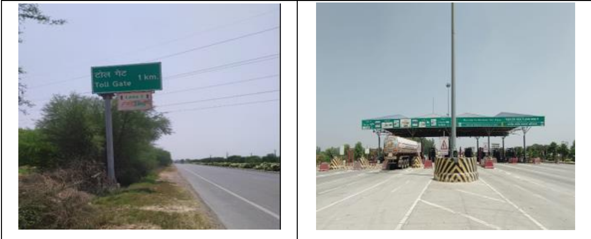
Figure 2-2 : Photographs showing Project Corridor
