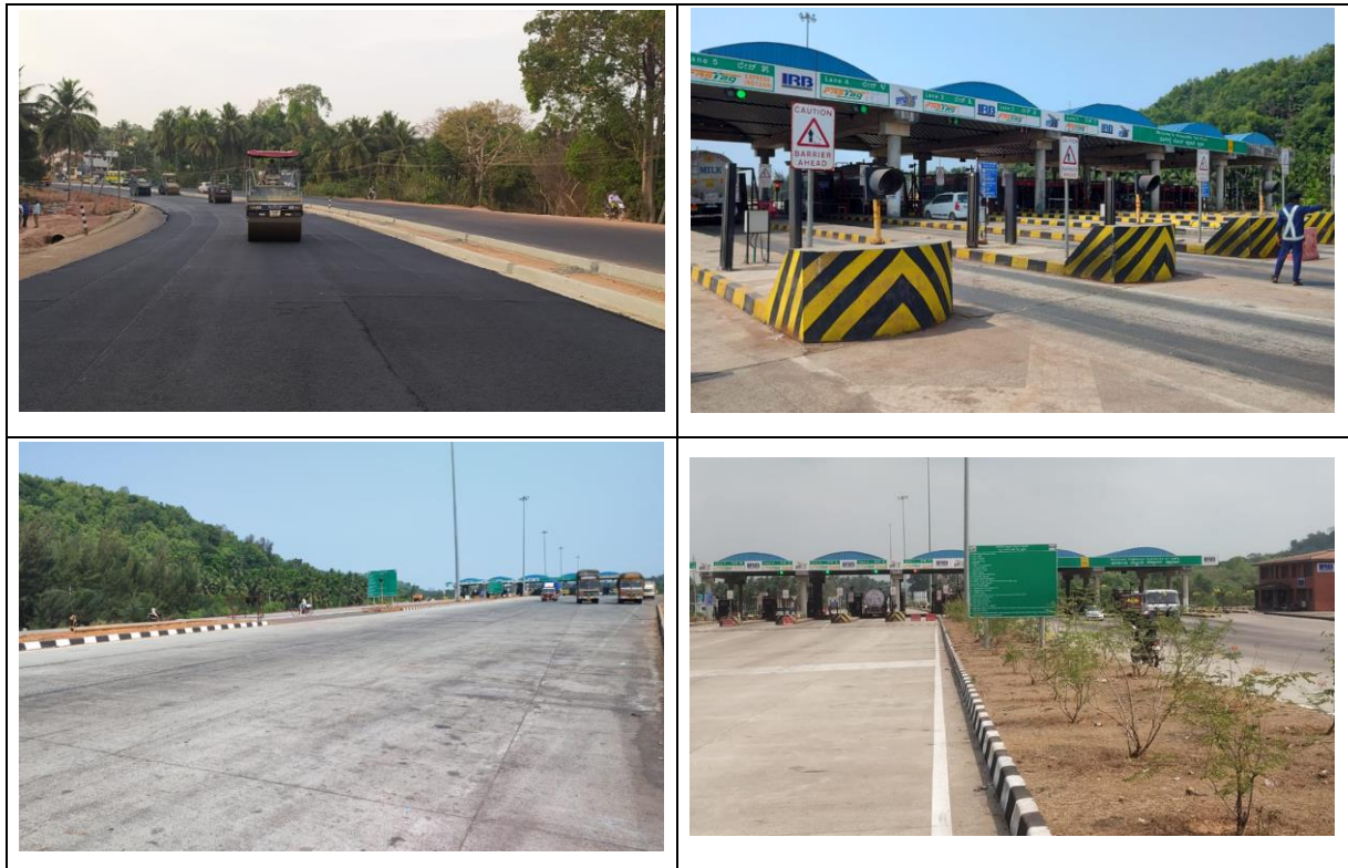
Figure 2-2 : Photographs showing Project Corridor
