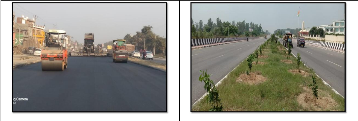
Figure 2-3: Photographs showing Project Corridor
