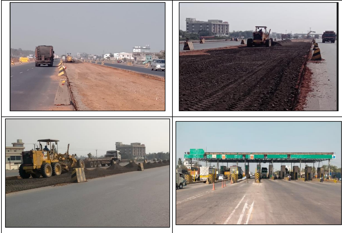
Figure 2-2: Photographs showing Project Corridor
