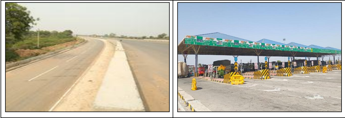
Figure 2-2: Photographs showing Project Corridor
