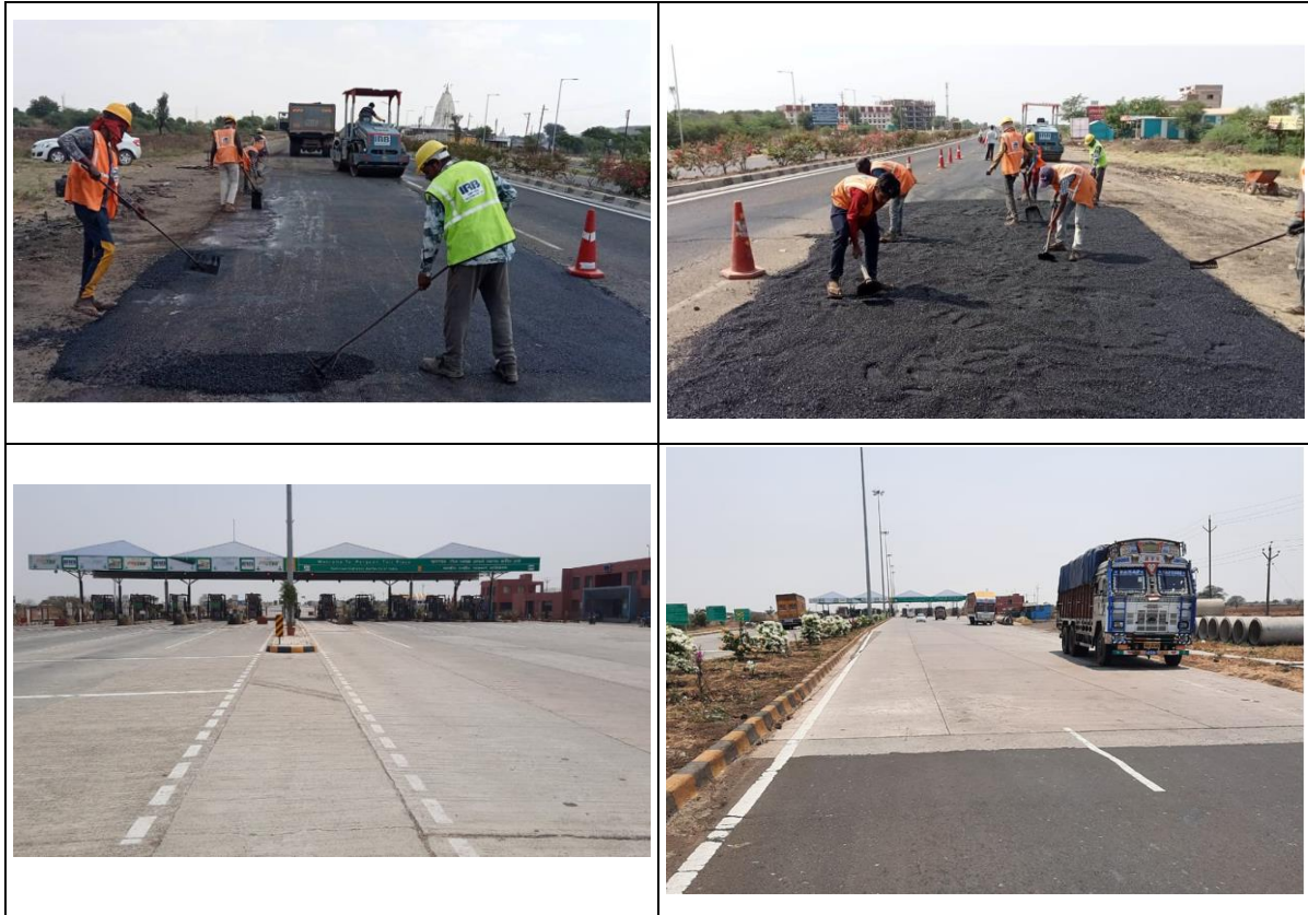
Figure 2-2 : Photographs showing Project Corridor
