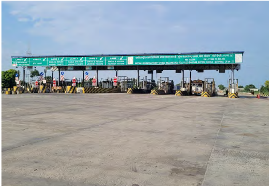
Figure 1-7 : Toll Plaza at Makhel
