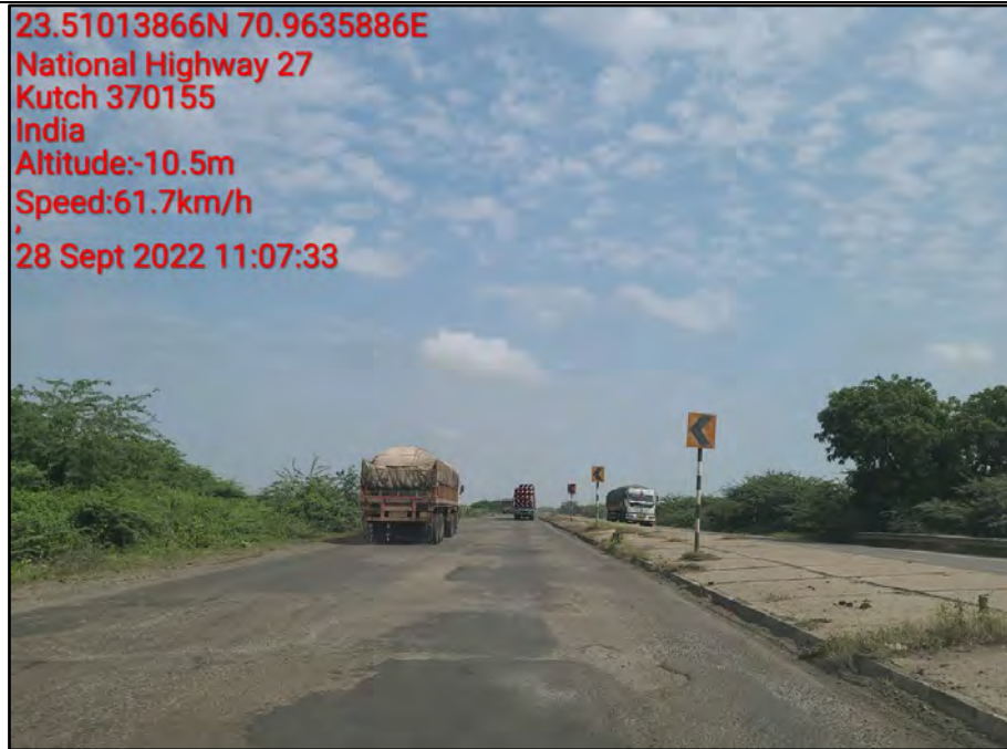
Figure 1-3 : Worn out wearing course of project road.
