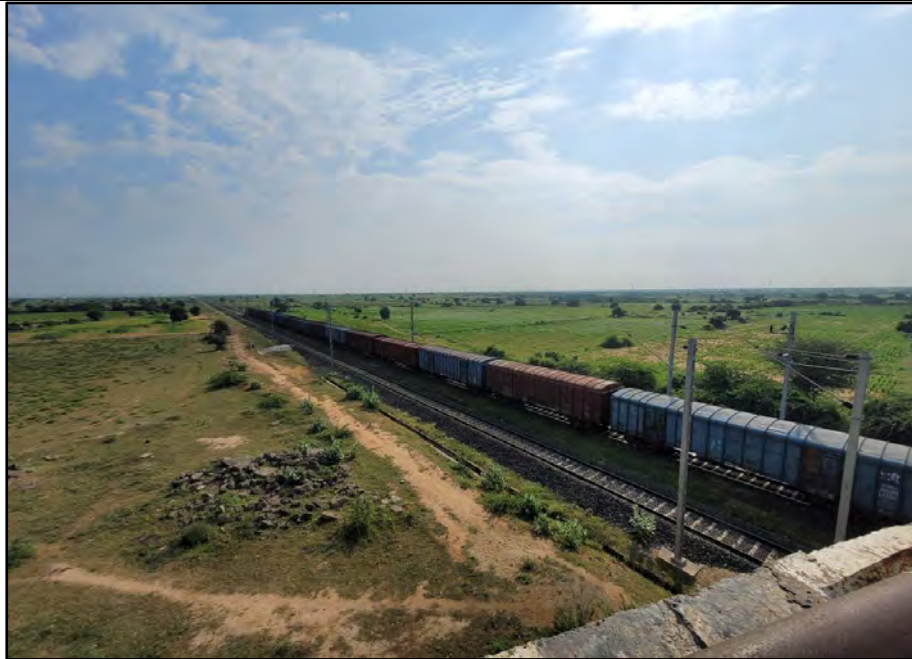
Figure 1-5 : Railway Line Palanpur- Kandla along Project Stretch
