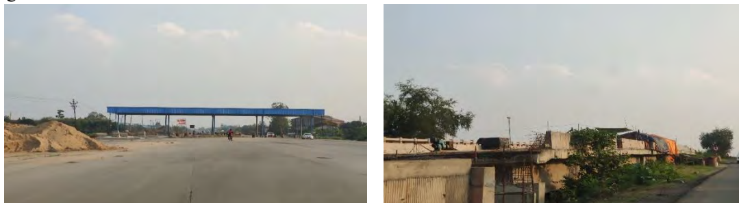
Figure 4-5 ROB & Toll Plaza under construction.
