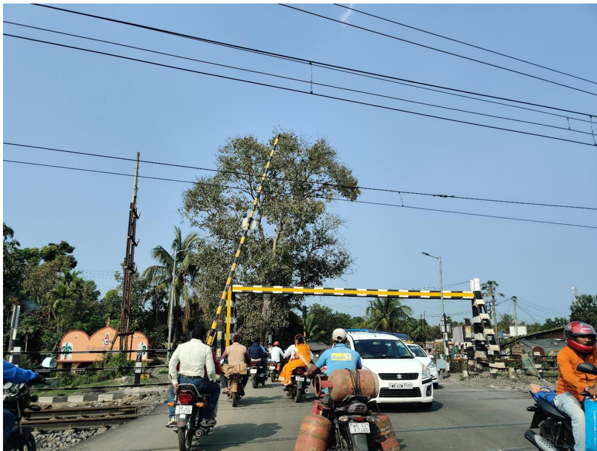
Figure 4-3 Railway level crossing at GT road.
