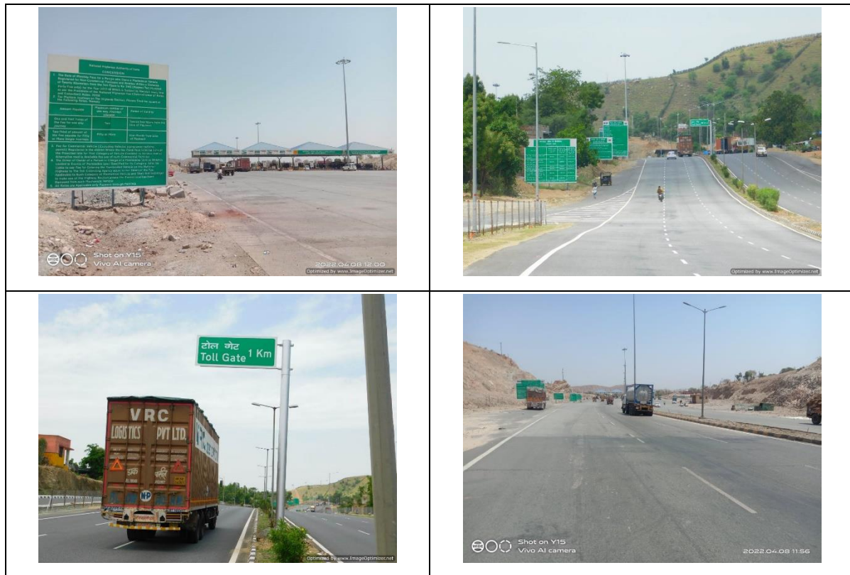
Figure 2-2 : Photographs showing Project Corridor
