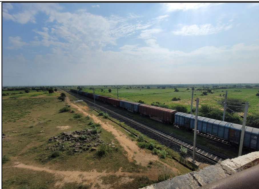
Figure 1-5 : Railway Line Palanpur- Kandla along Project Stretch
