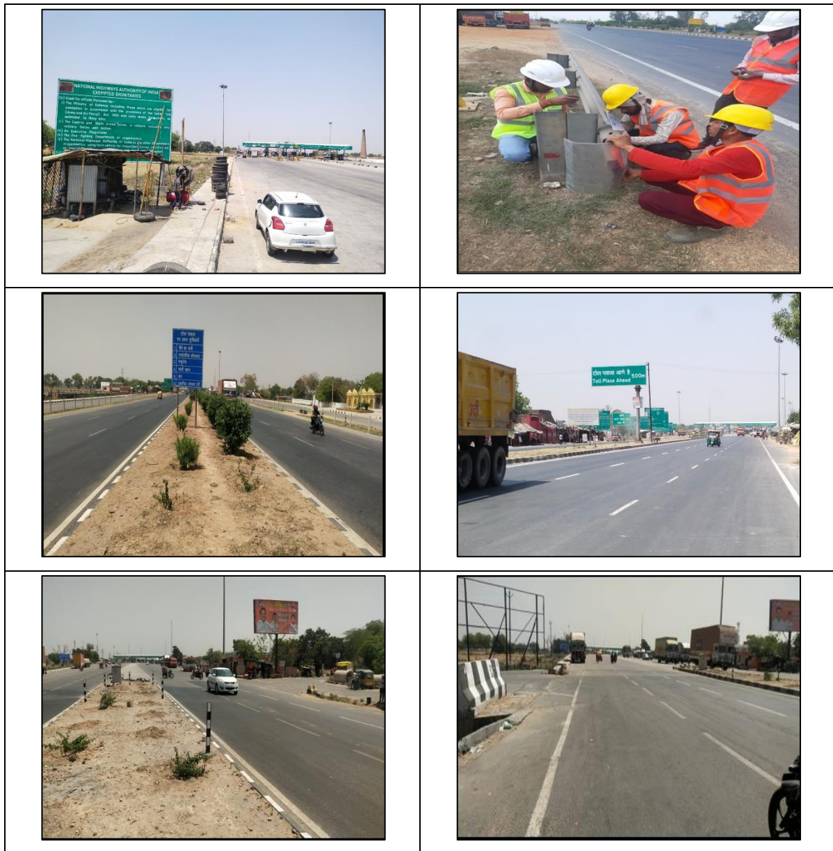
Figure 2-2: Photographs showing Project Corridor
