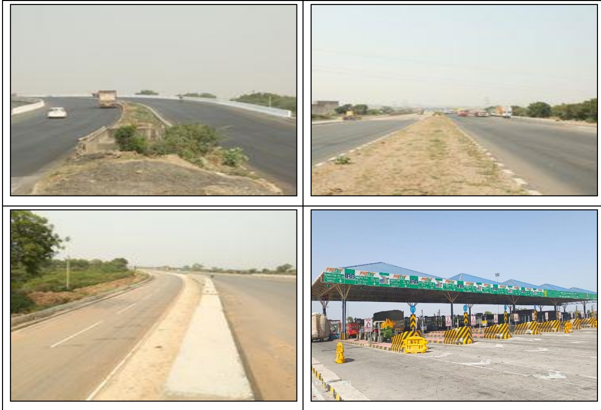
Figure 2-2: Photographs showing Project Corridor
