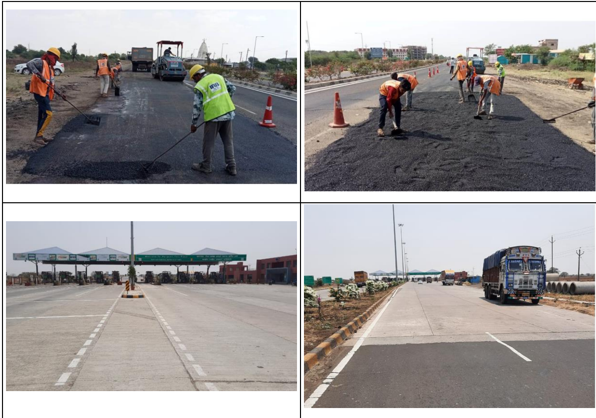
Figure 2-2 : Photographs showing Project Corridor
