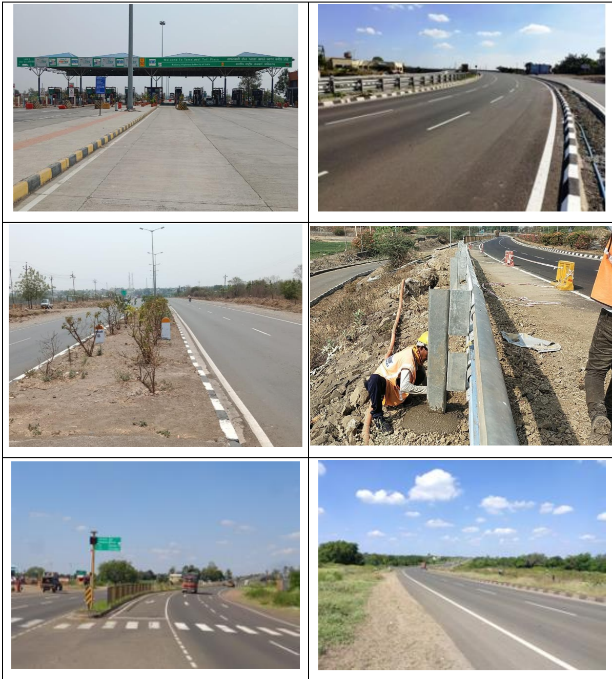
Figure 2-2: Photographs showing Project Corridor
