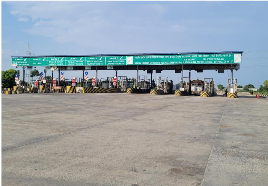
Figure 1-7 : Toll Plaza at Makhel
