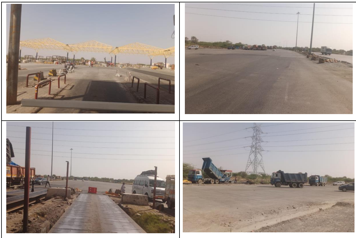
Figure 2-2 : Photographs showing Project Corridor
