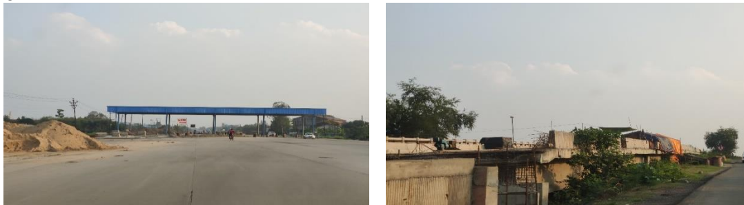
Figure 4-5 ROB & Toll Plaza under construction.
