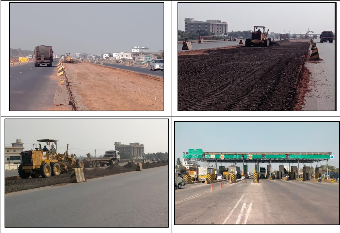
Figure 2-2: Photographs showing Project Corridor
