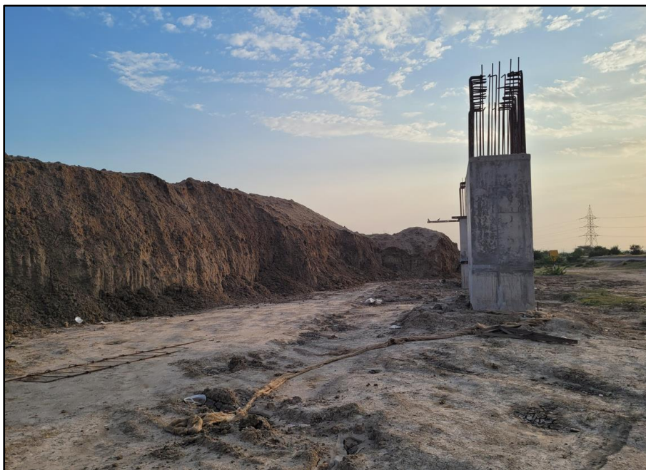
Figure 1-6 : Interchange at connection of Amritsar – Jamnagar Expressway near Santalpur
