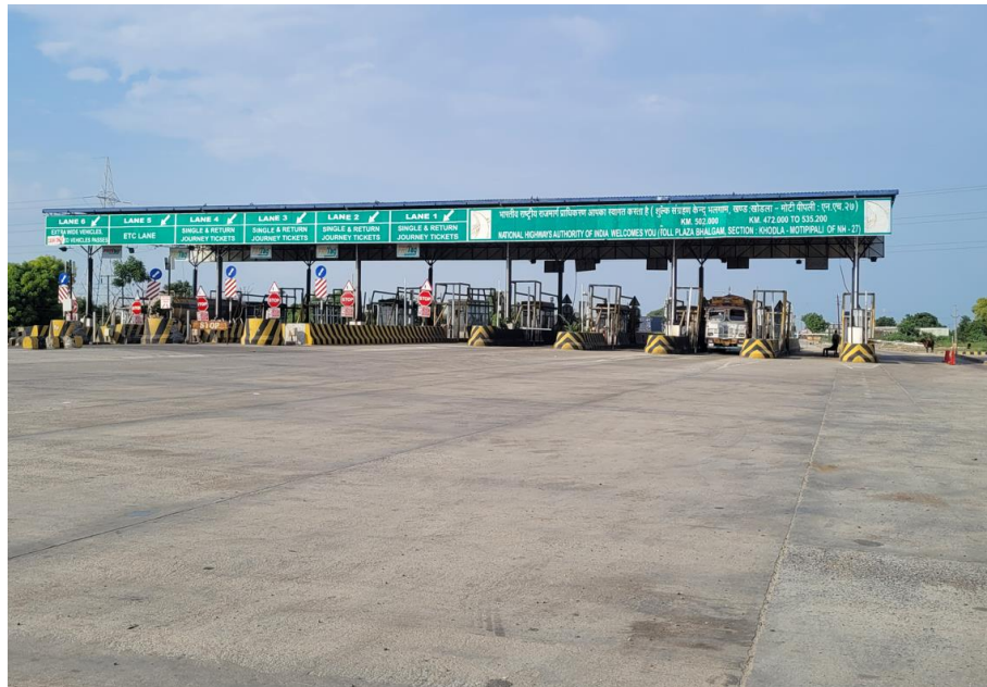
Figure 1-7 : Toll Plaza at Makhel
