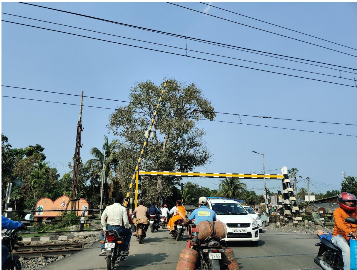
Figure 4-3 Railway level crossing at GT road.
